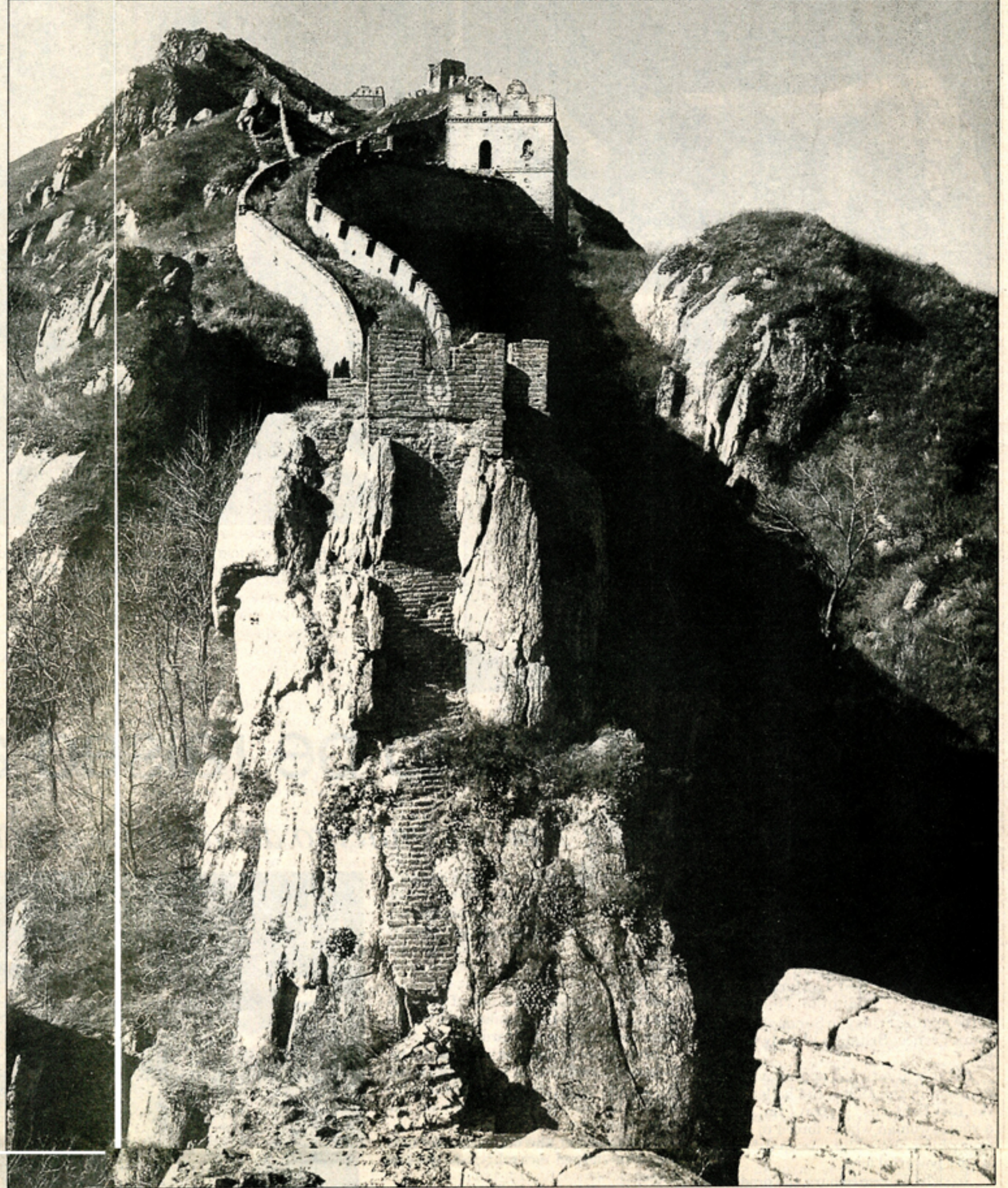
Cliffside view: A segment of the wall on the east side of Badaling which is not open to tourists. Though part of the wall has collapsed, people can still see how centuries ago builders used the rocks on the mountains as a natural part of the wall, and chose steep terrain for the erection of forts.
