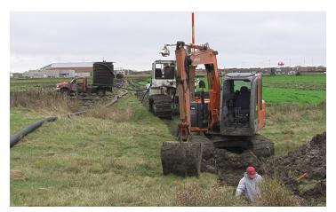
A lot of equipment is required to install tile drainage.
