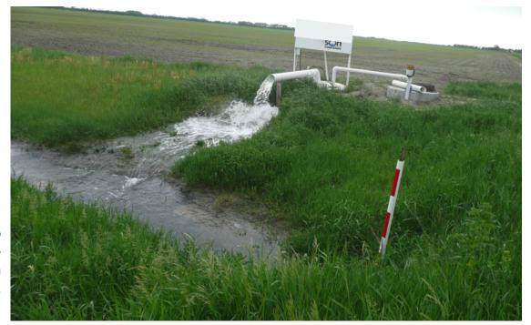
Drainage pump station discharge mixes with surface runoff.
