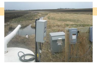
Pumped outlets increase the initial investment and operation/maintenance costs of the tile drainage system but may be economically feasible in many situations. A pumped outlet station includes a sump, pump, discharge pipe and usually an electric control panel. Important design features include the storage volume of the sump and capacity (flow rate) of the pump.
