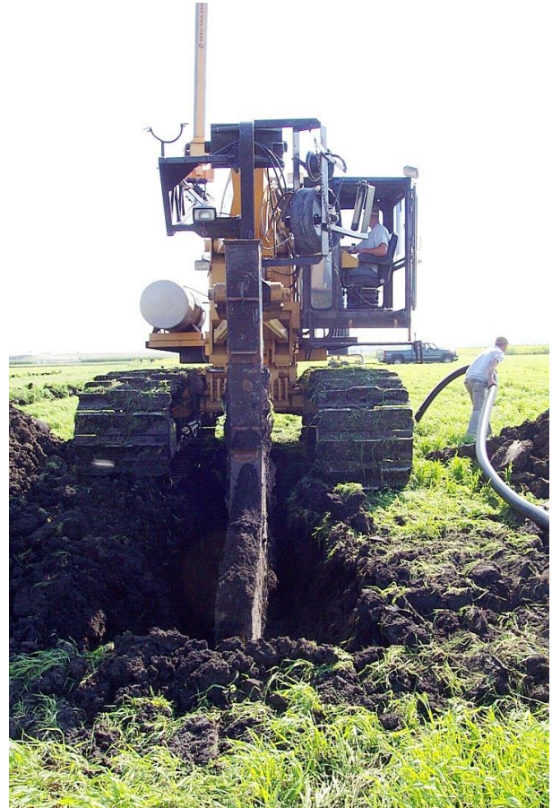
Photo: Installing subsurface drain tile.
