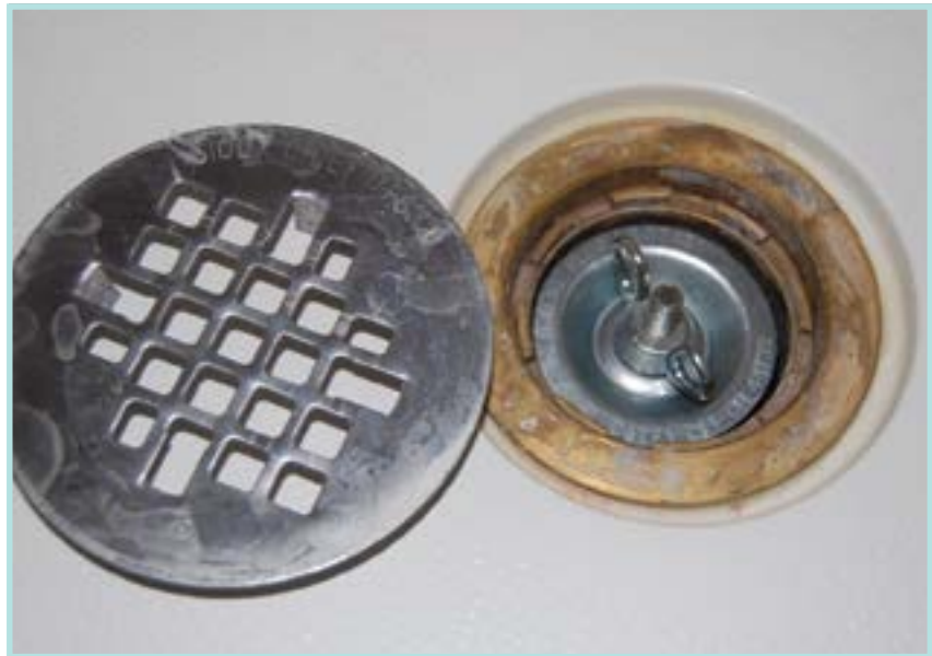
Figure 14. Plugging shower drain.
