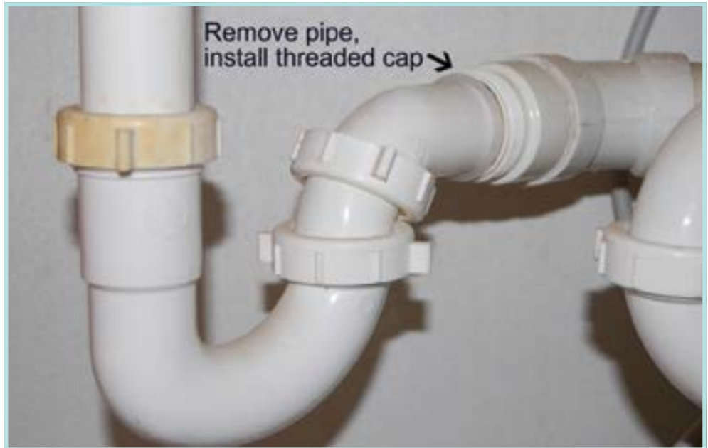
Figure 16. P trap under sink.
