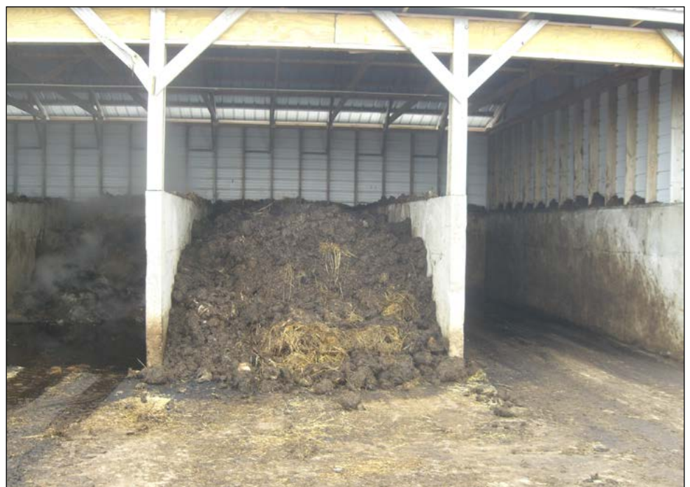
Figure 2. Bins arranged for sow and litter composting. Additional space is for co-composting material storage and handling. (NDSU photo)
