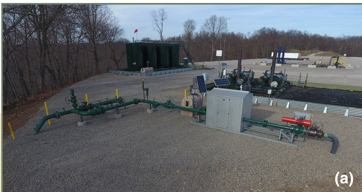
Figure 10. (a) Pipelines on a well pad (Harold Rhodes) and (b) an example of a tanker truck used to transport both fresh water and brine water (Sam Croat).
