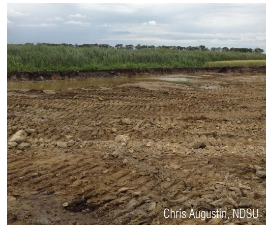
Figure 6. The topsoil was removed from this spill site as part of ex situ remediation.
