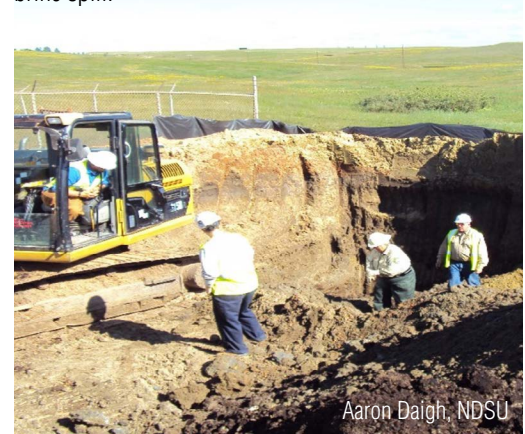
Figure 5. A crew is doing ex situ remediation of a brine spill.
