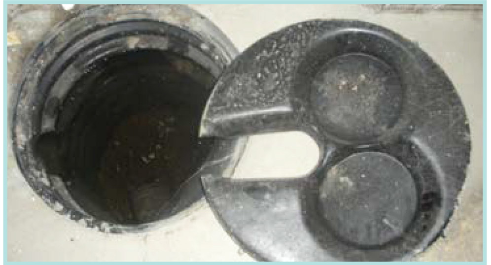
Figure 19. Footing drain.
