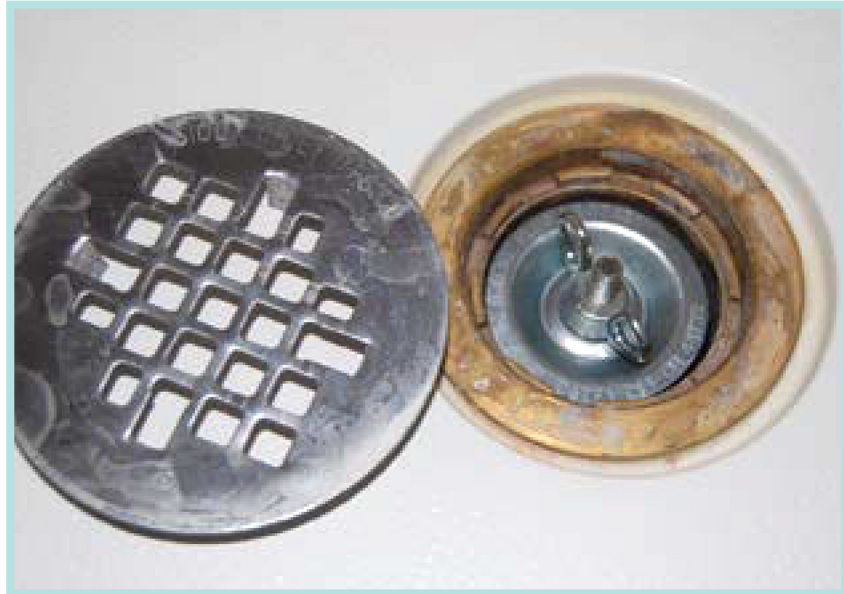
Figure 14. Plugging shower drain.
