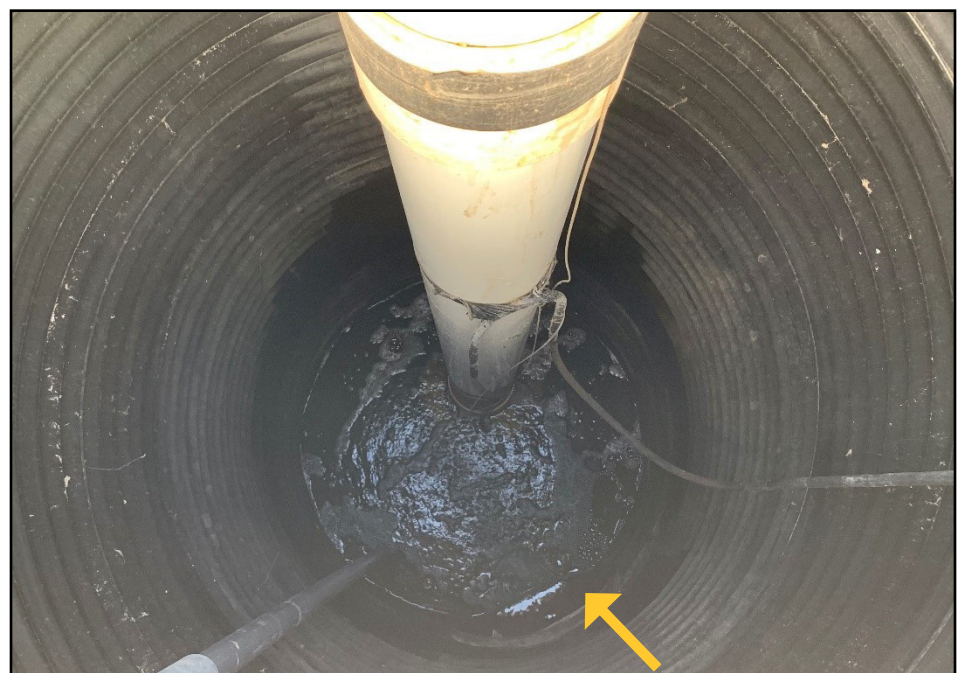
Figure 6. This submersible pump at the NDSU Langdon Research Extension Center's tiled research site is not pumping water despite standing water at a low spot on Sept. 13, 2019, due to the poor soil water infiltration resulting in reduced drainage performance. The main drain is indicated by the arrow. (N. Kalwar, NDSU)
