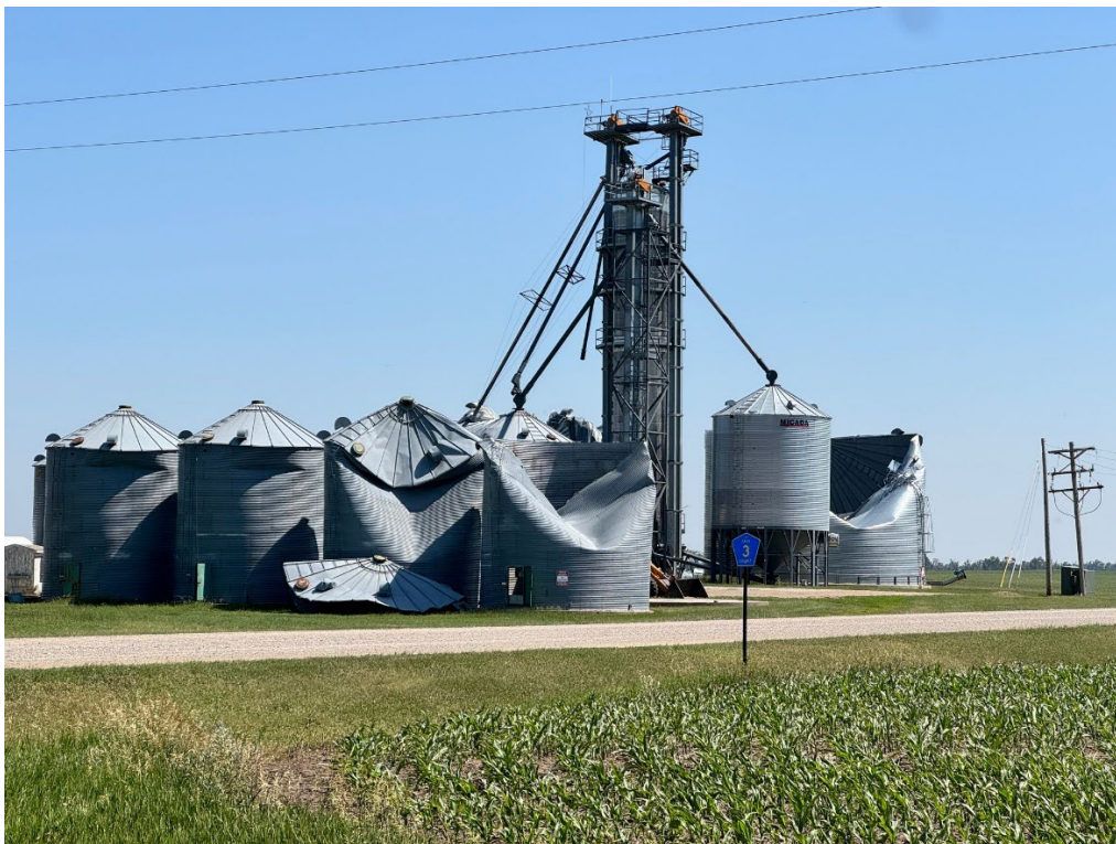
Damage to grain bins to the east of Pillsbury, North Dakota associated with the with the extreme long-lasting wind that moved through that area. (photo courtesy of Daryl Ritchison)
