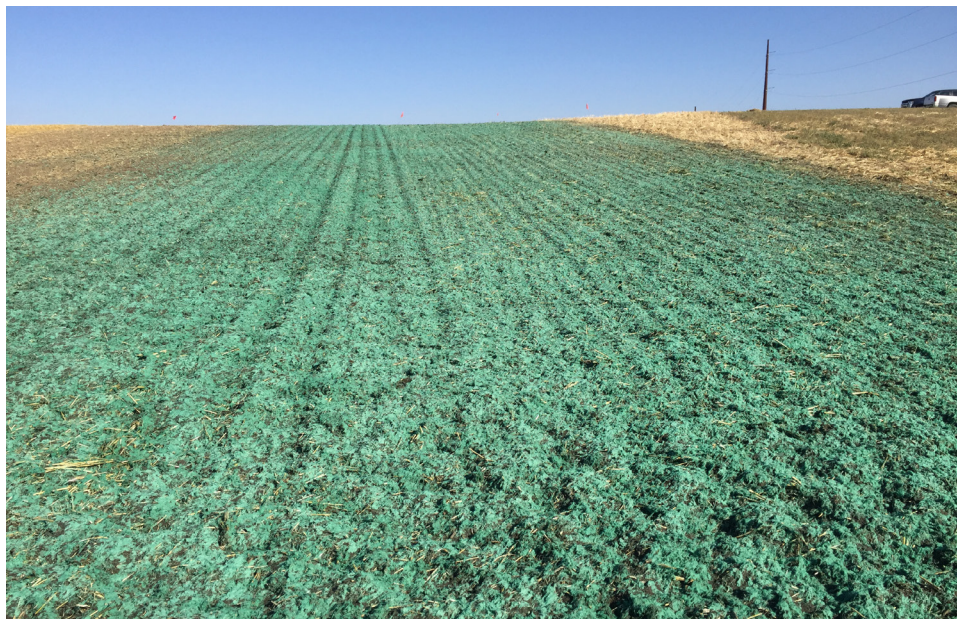
Hydromulch used to stabilize a disturbed site.
