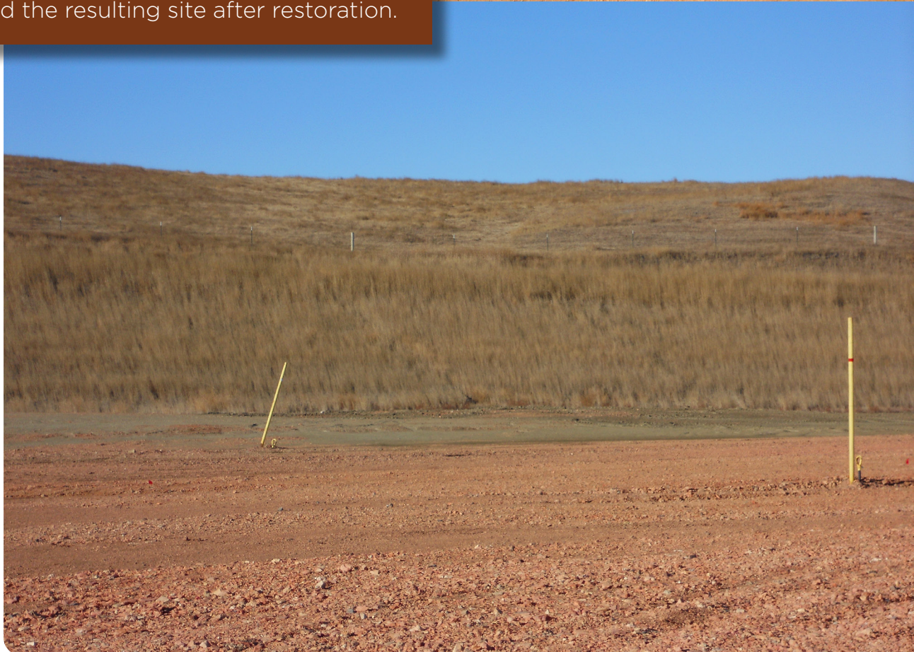
Final restoration with erosion control structures removed
