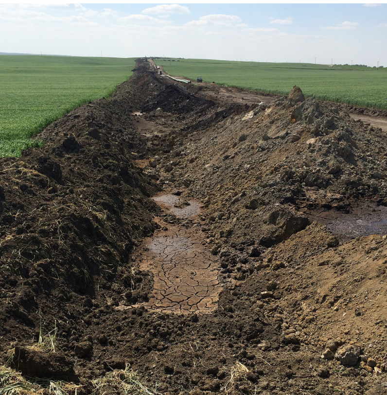
Separation of topsoil and subsoil during pipeline installation.
