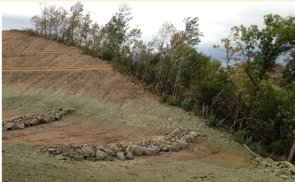
Site utilizing multiple erosion control methods to reduce sediment loss.
