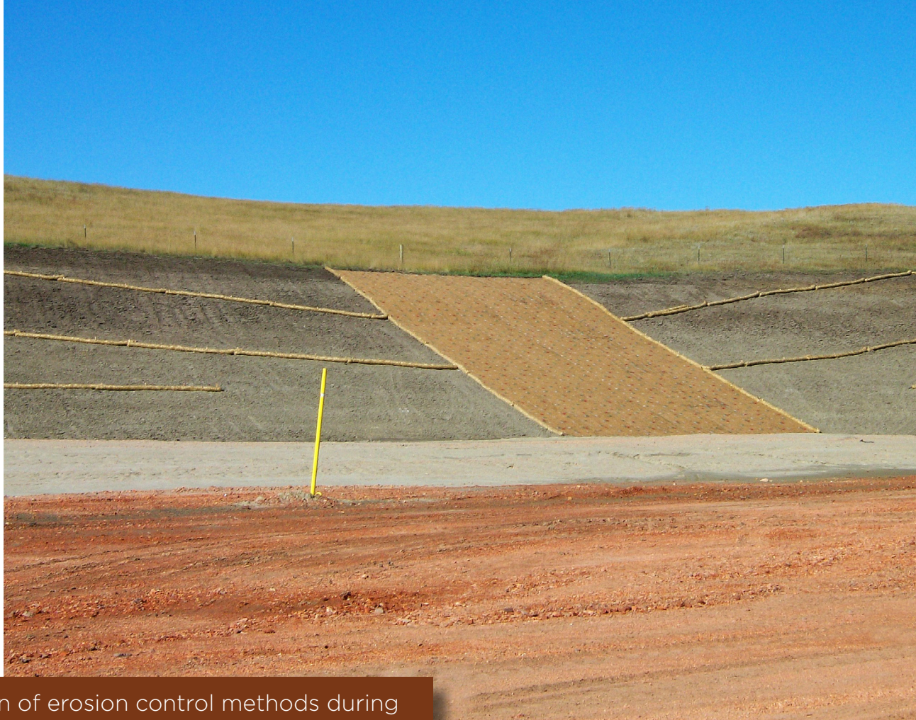
Erosion control during the reclamation process
