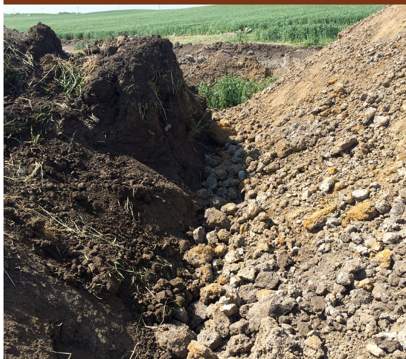
Separation of topsoil and subsoil during pipeline installation.
