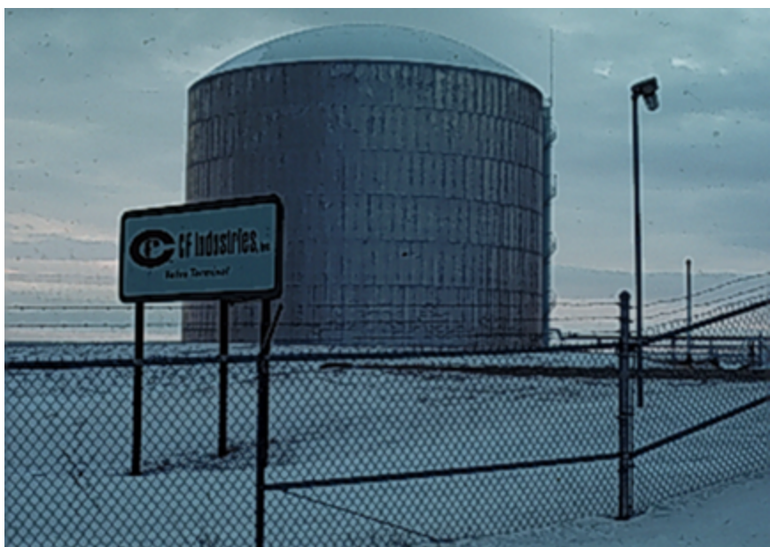
Figure 15.8 Large ammonia storage facility near Leal, ND with internal temperature regulated to about -28F, with resulting pressure less than 1 psi
