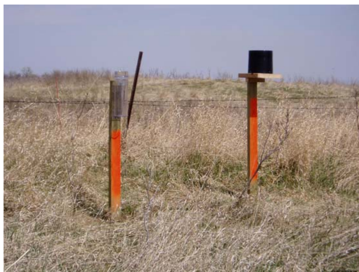
Figure 4 Installation of manual and tipping bucket rain gauge
