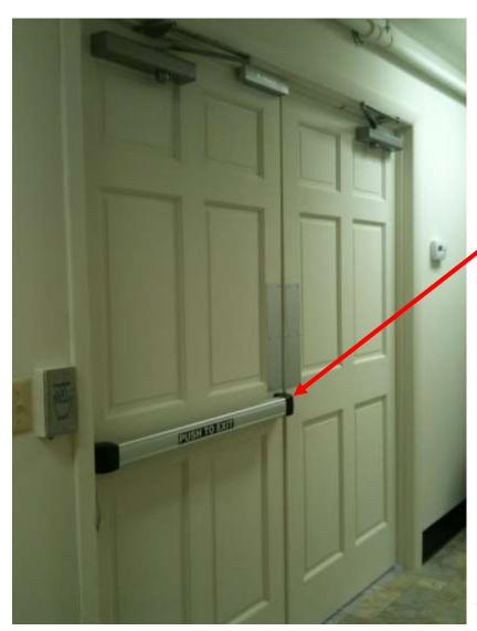
If there's enough room, a piece of copper wire inserted through door frame and touched to bar will trigger sensor.
