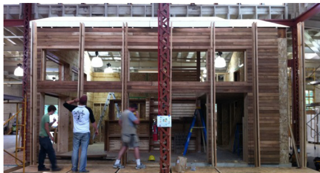
Students install verticals for shading structure.
