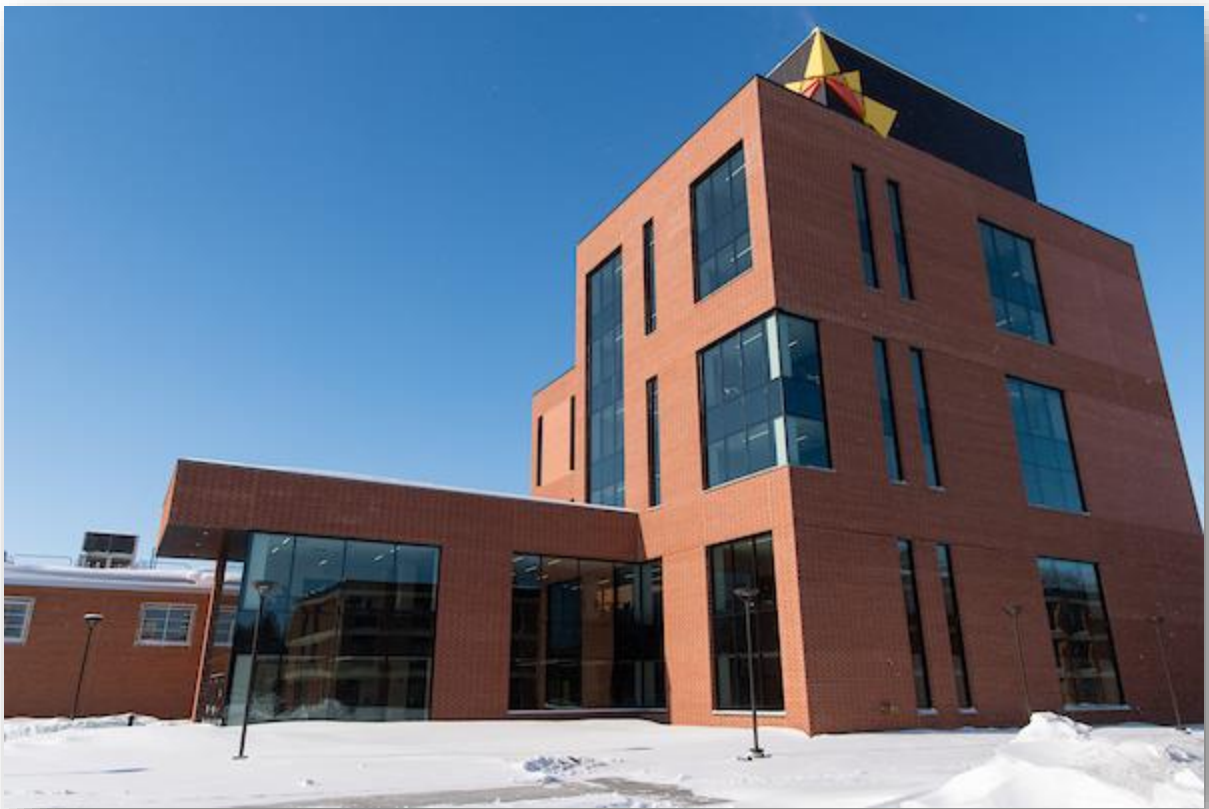
NDSU's Aldevron Tower - the Department of Public Health is on the 6th floor Image Source: https://www.ndsu.edu/alphaindex/buildings/Building:454
