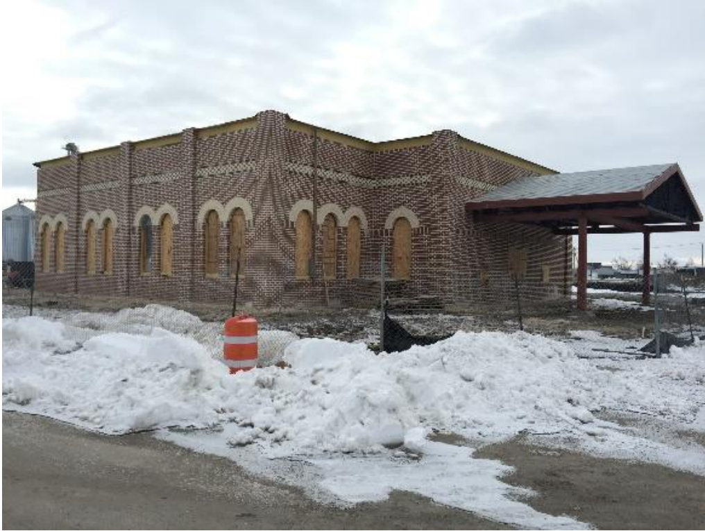
Photograph 5. Midwest Bank Construction. Source: Kurt Mantonya
