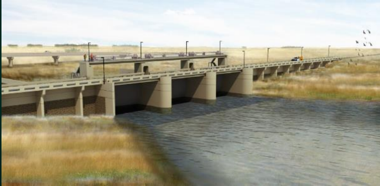
FM Flood diversion
