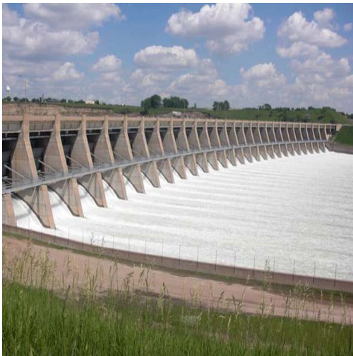
Garrison dam spillways
