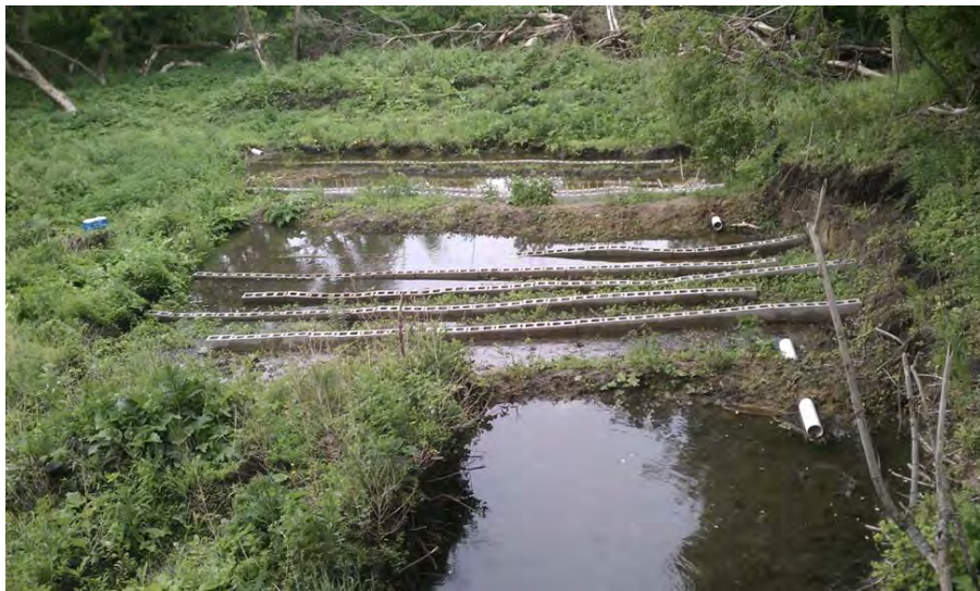
The constructed wetland at the Embden Discovery Farm (May 2012). The system was constructed in 2011. The emergent helophytes, cattails ( Typha latifolia ), have yet to emerge. The banks of the system host fast-growing willow (a hybrid known as QC83, which grows 3 m/yr) for production of biogasification fuel (photo by Alex Stalboerger).
