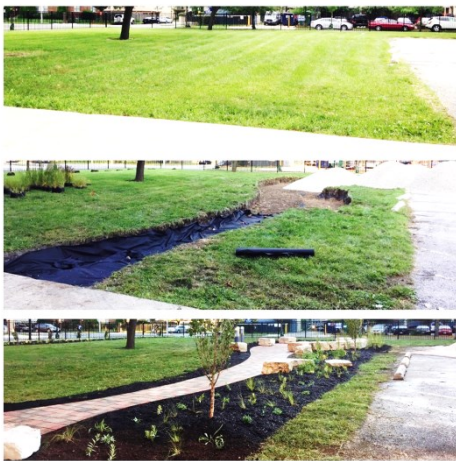
Rain garden construction progress at Pershing Magnet School Chicago, IL. Photo courtesy of the Metropolitan Water Reclamation District of Greater Chicago.
