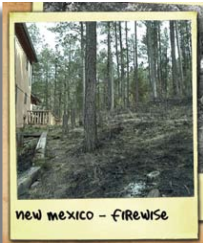
Fire burned very close to this home in New Mexico without igniting the wood walls.
