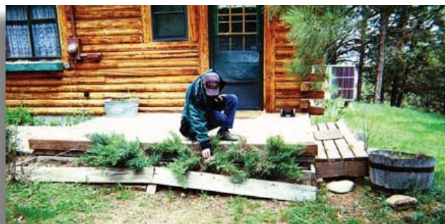
Flammable vegetation in direct contact with house
