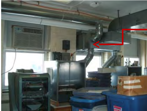
Inadequate, temporary ventilation added to research lab
