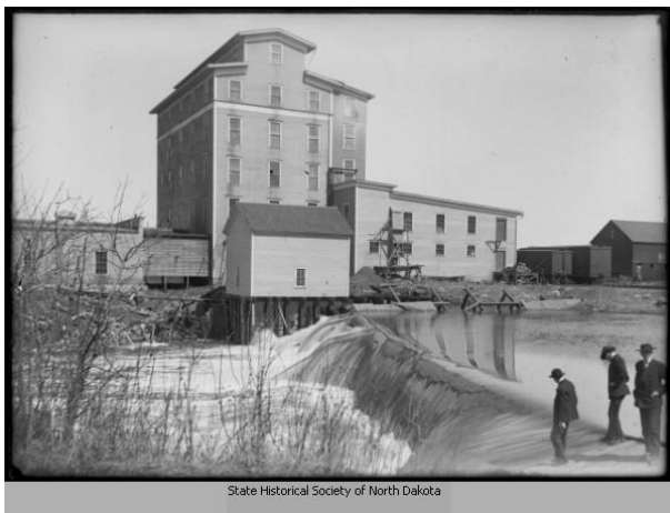
Photograph 3.1 Russell Miller Milling Company Source: Used by Permission, digitalhorizonsonline.org
