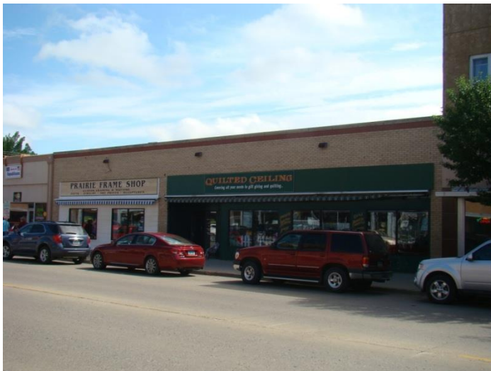
Photograph 3.3. Quilted Ceiling, Valley City, 2012
