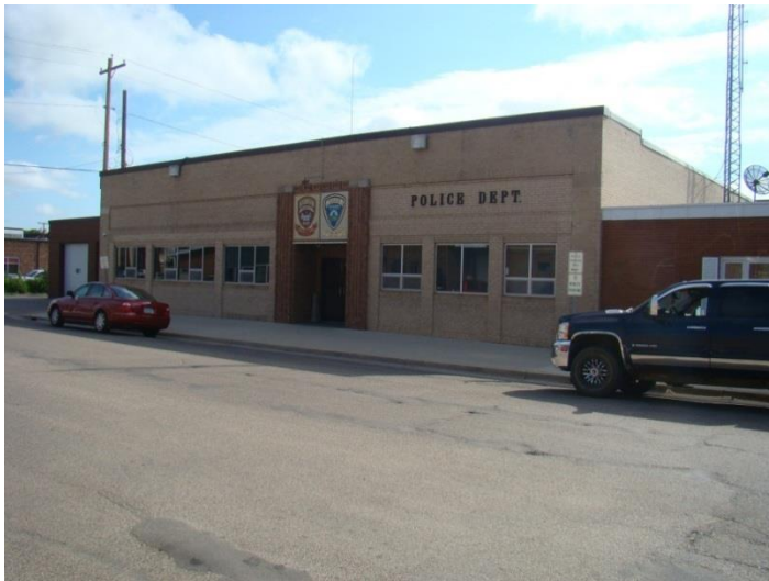
Photograph 10.3 Valley City Police Department
